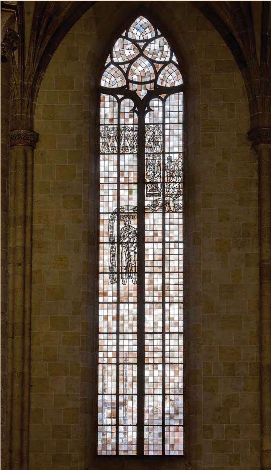
1 Bestandsfenster Yelin in Fensterposition nXI.
